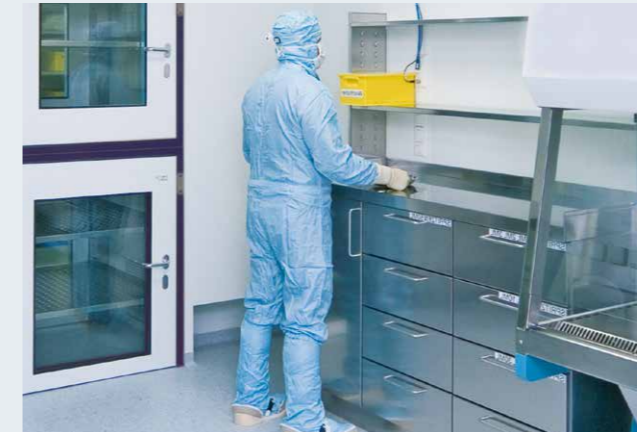
Individual clean room equipment with cytostatic safety cabinet, insulator technology and material airlocks
